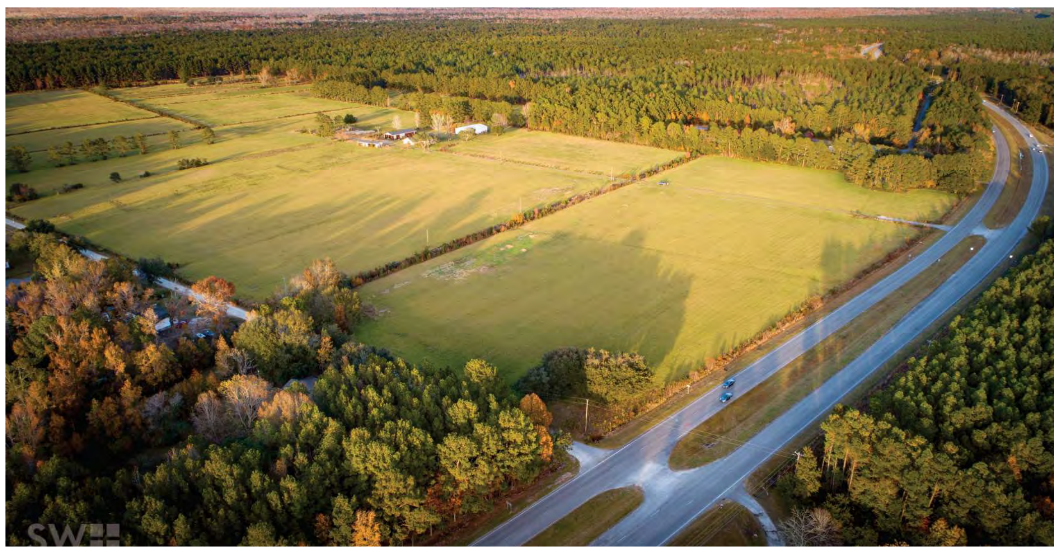
1 VIEW LOOKING NORTHEAST AT SITE FROM HWY. 17
